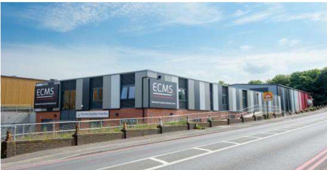
The Elite Centre for Manufacturing Skills National Foundry Training Centre in Tipton.
